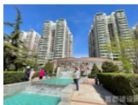
“首开经验”助力老旧小区...
